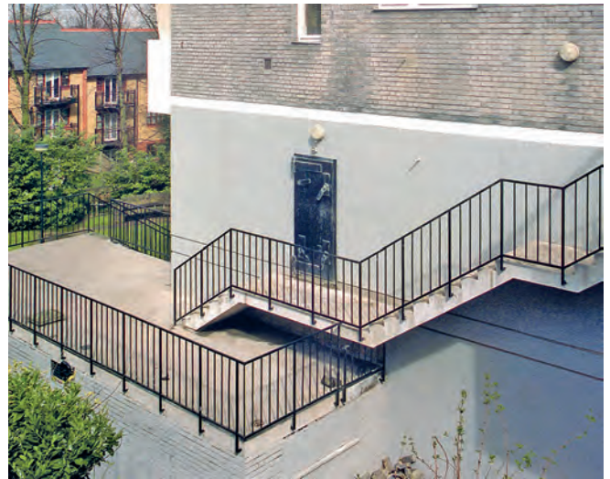
Blast door into the upper floor of the Pear Tree House bunker in 2001. Photo Nick Catford
